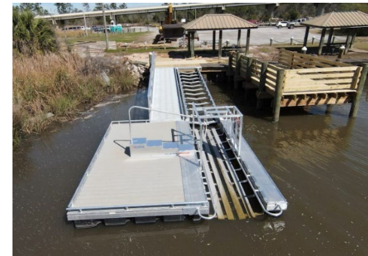
ADA Platform with Transfer Station
