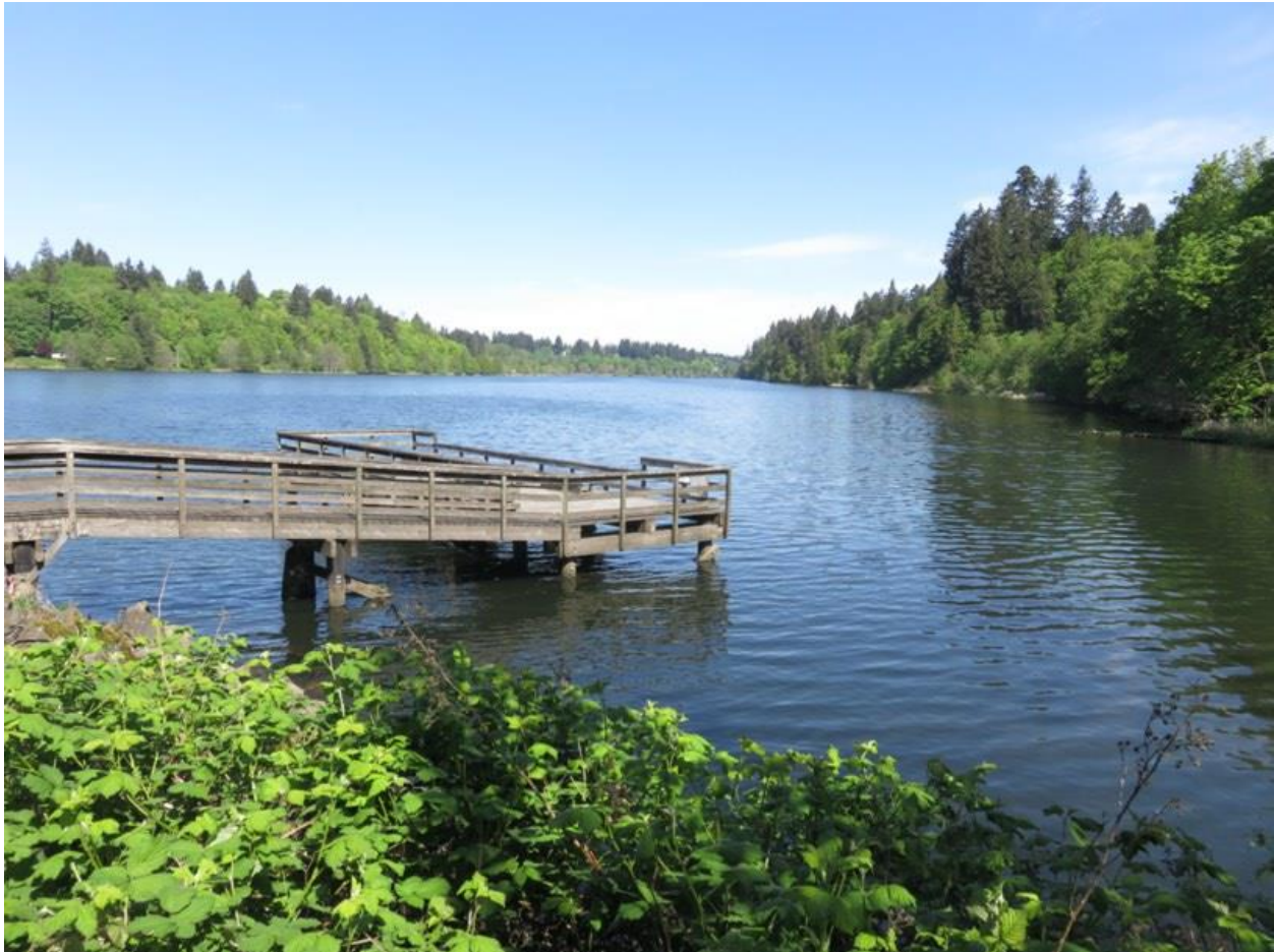
Photo 9 Interpretive Center pier looking north
