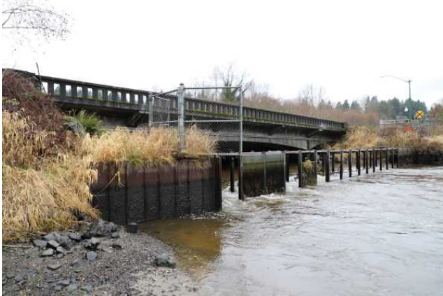
Bridge, southeast corner.
