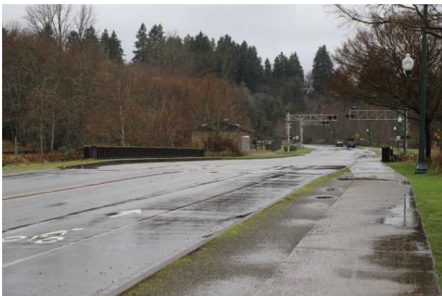
Road deck looking north.
