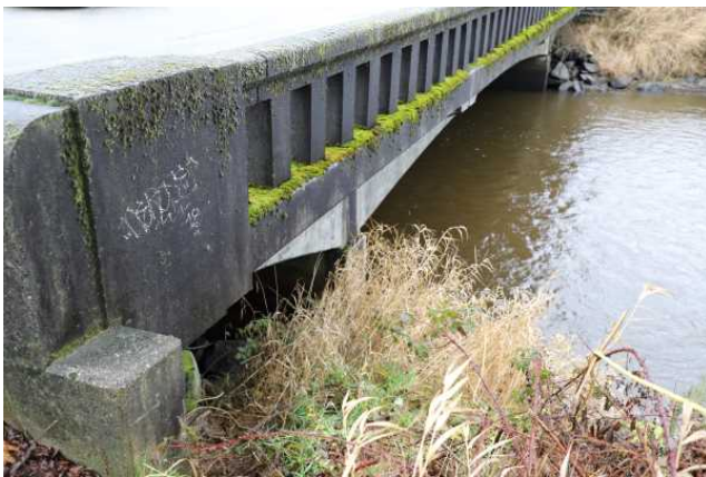
Bridge structure, detail.
