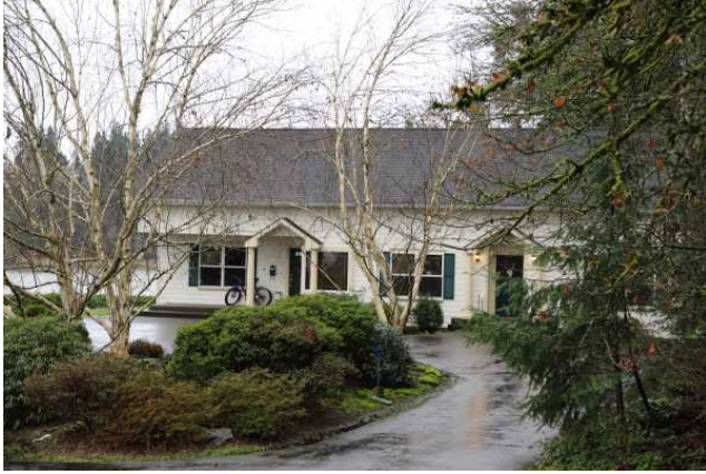
North facade detail.
