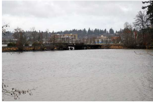
Bridge, south side (1)
