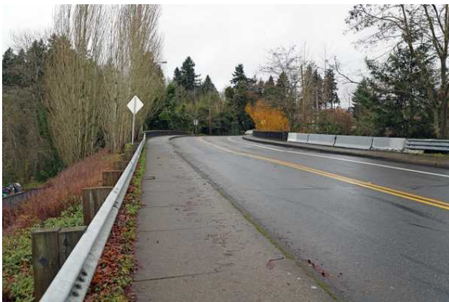
Guard rails and jersey barriers. (8)
