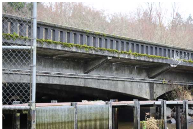
Bridge structure, detail.
