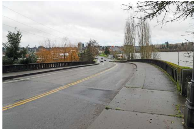
Span and associated guard rails. (11)
