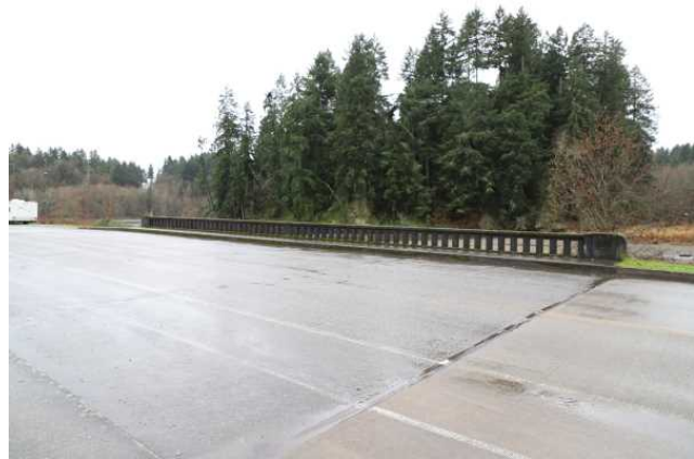
Railing, looking southwest.
