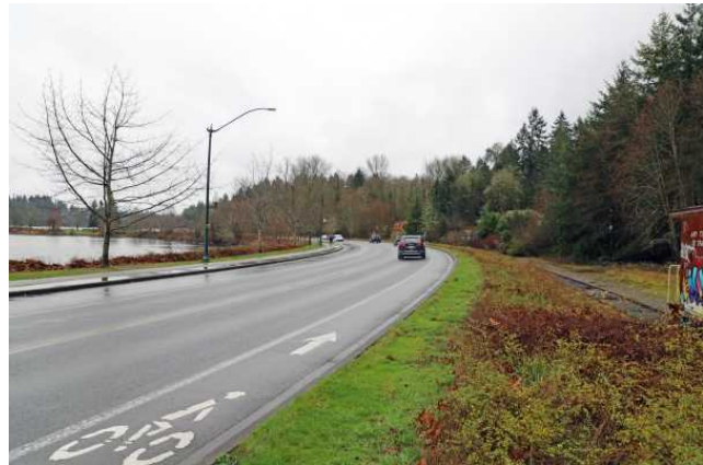
Shoulder and former railway conditions along the west side of the parkway. (9)
