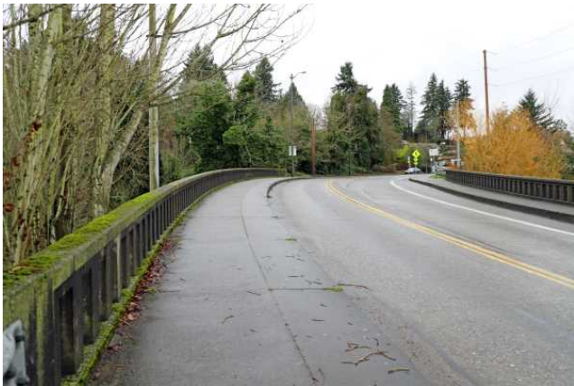
Span looking west. (10)
