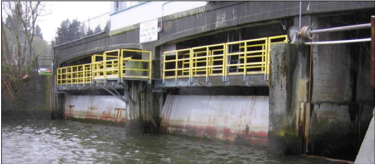
Figure 2-31 Photograph of 5 th Avenue Dam Looking Northward (M&N 2008)
