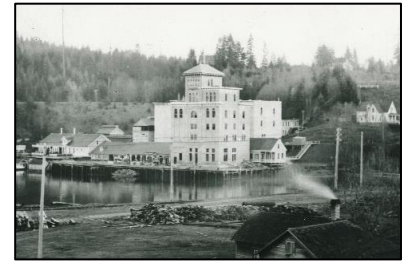
Exhibit 4.10 Undated black and white photo of the Brewery Building and powerhouse. (Source: State Library Photograph Collection, 1851-1990, Washington State Archives. Original images held at the Washington State Archives, Olympia, WA)
