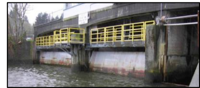
Exhibit 3.2 View of the 5 th Avenue Dam from the North Basin
