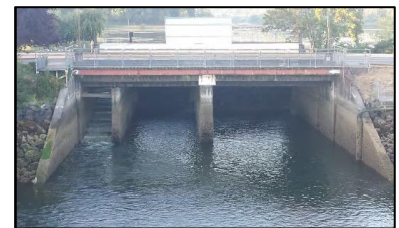
Exhibit 3.16 Fish ladder at 5 th Avenue Dam, at left
