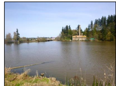
Exhibit 3.48 Steam plant on the northeast shore of the Middle Basin
