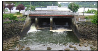
Exhibit 2.13 Existing tide gates at 5 th Avenue Dam (Source: Moffatt & Nichol)
