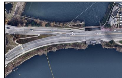
Exhibit 2.14 Earthen portion of 5 th Avenue Dam
