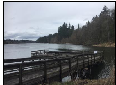
Exhibit 2.7 View of dock at the southern point of the Interpretive Center
