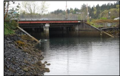
Exhibit 2.17 Riprap along the shoreline near the existing 5 th Avenue Bridge
