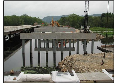
Exhibit 2.11 Bridge pile bent (Source: Federal Highway Administration)
