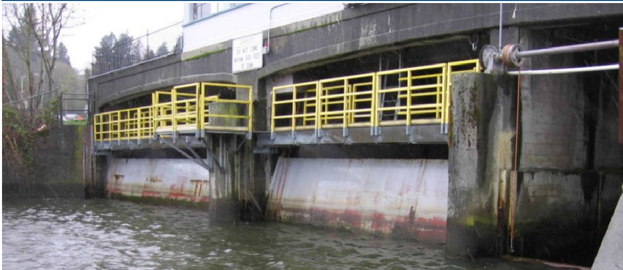
Figure 3.4 Photo of the 5 th Avenue Dam Looking North from Upstream
