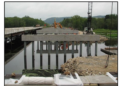
Bridge pile bent (Source: Federal Highway Administration)
