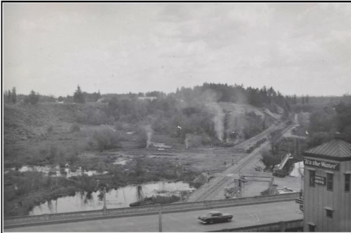
Here, an unknown photographer stood on the roof of the modern Olympia brewery and took a picture of the valley to the southeast. In 1953, the brewery was preparing to expand into this area—the first steps were clearing the site and filling in the marsh to provide solid footing for the large buildings to come.
