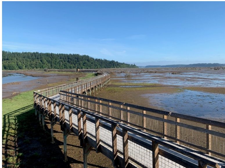
Boardwalks similar to this one at the Nisqually National Wildlife Refuge would be constructed in the Middle and South Basins under all of the action alternatives
