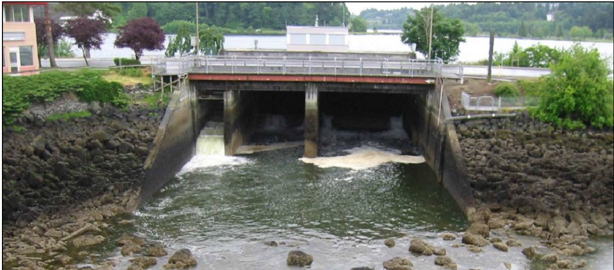
Figure 2-30 Photo of the North Side of the 5 th Avenue Dam Looking South (M&N 2008)
