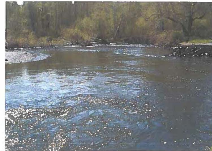
Heavy Erosion, High Risk to Floaters, 4/20/17
