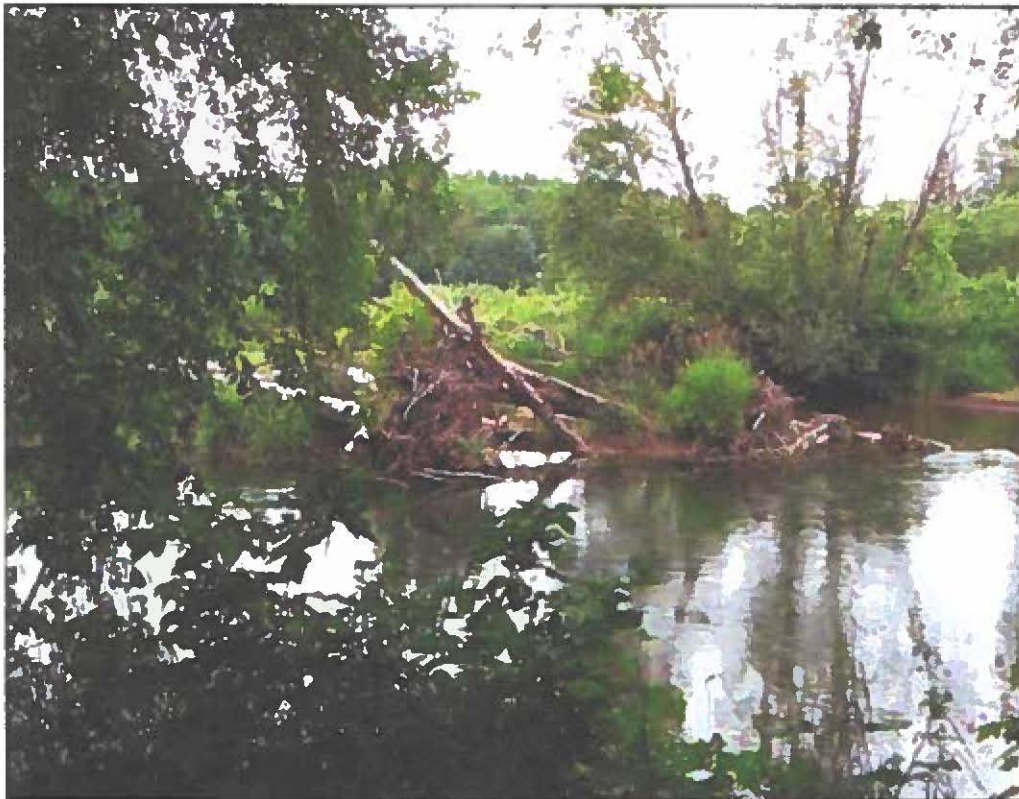
Log structure and rock W-veins direct flow to center of the river
