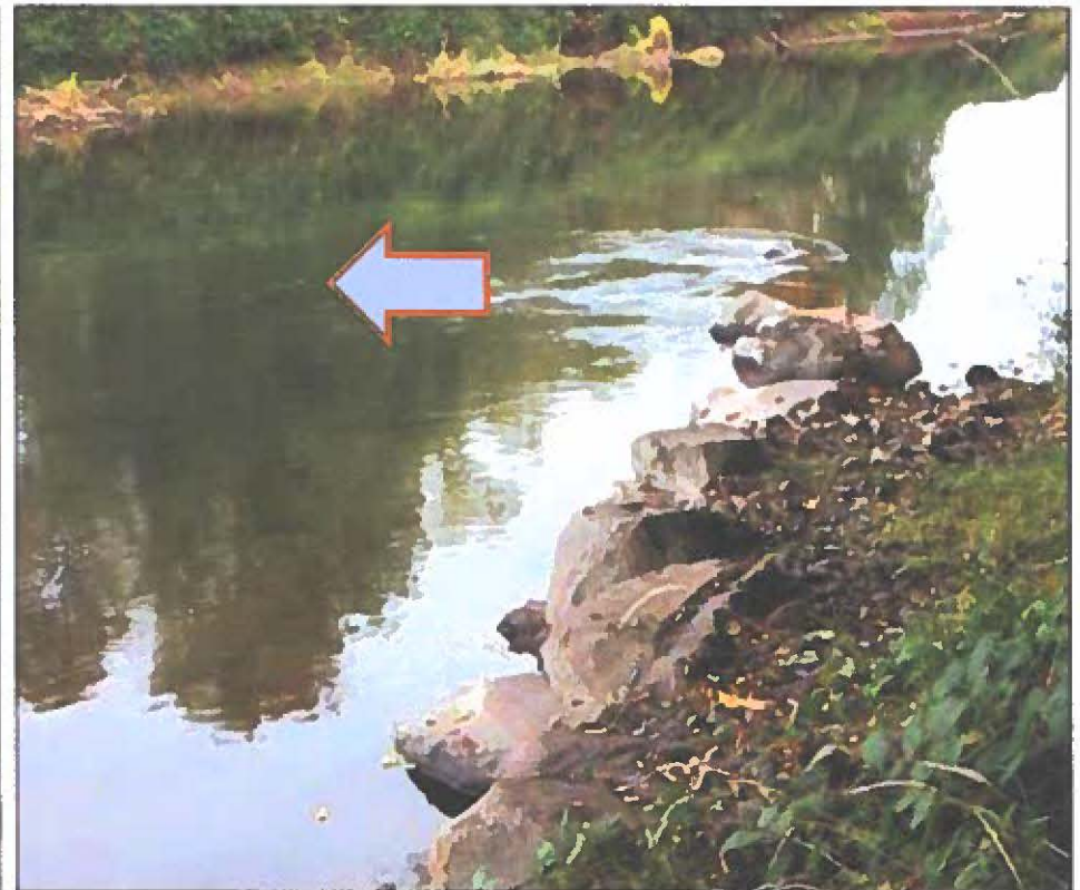
Rock J-hooks direct flow away from bank
