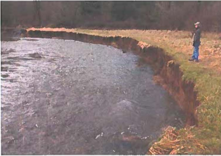
Heavy erosion at Pioneer Park 1/10/16.
