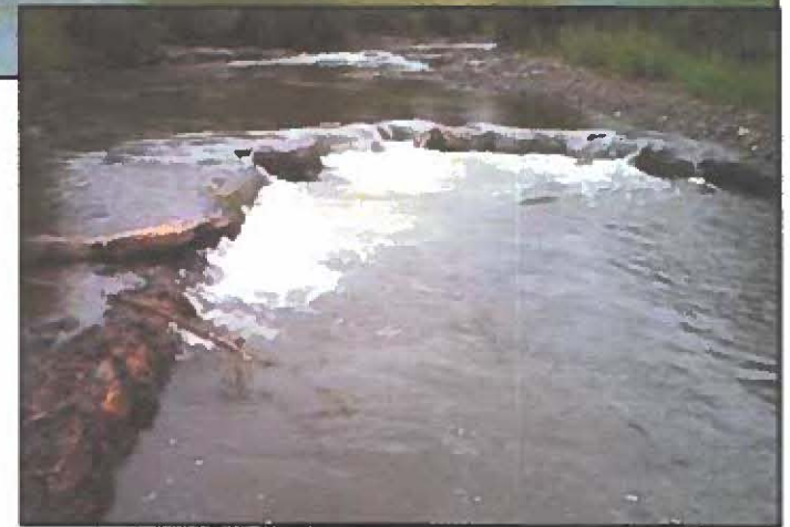
Wood rock crossvanes provide deep water habitat
