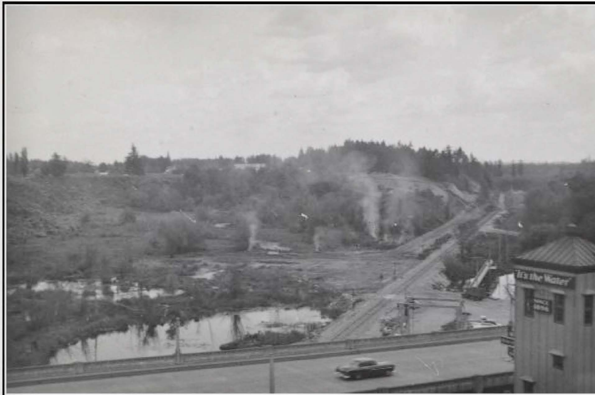
Here, an unknown photographer stood on the roof of the modern Olympia brewery and took a picture of the valley to the southeast. In 1953, the brewery was preparing to expand into this area—the first steps were clearing the site and filling in the marsh to provide solid footing for the large buildings to come.
