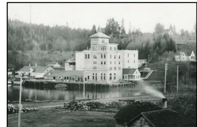
Exhibit 4.83 Undated black and white photo of the Brewery Building and powerhouse. (Source: State Library Photograph Collection, 1851-1990, Washington State Archives. Original images held at the Washington State Archives, Olympia, WA)
