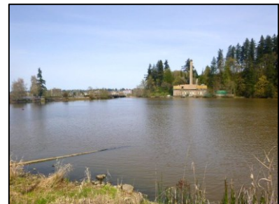
Exhibit 3.69 Steam plant on the northeast shore of the Middle Basin
