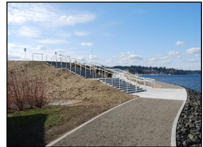
Exhibit 3.71 NorthPoint on the Port Peninsula
