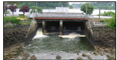
Exhibit 2.17 Existing tide gates at 5 th Avenue Dam (Source: Moffatt & Nichol)
