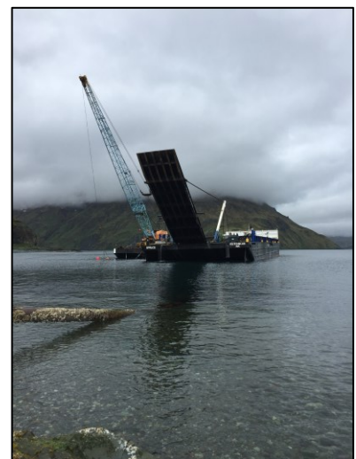
Exhibit 2.23 Images of a mechanical dredge
