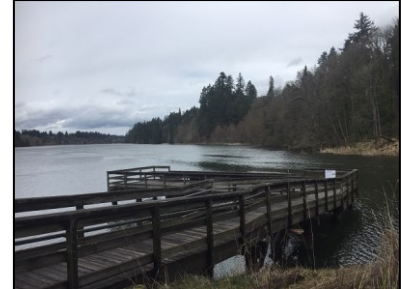
Exhibit 2.11 View of dock at the southern point of the Interpretive Center
