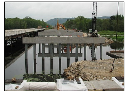
Exhibit 2.15 Bridge pile bent (Source: Federal Highway Administration)
