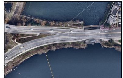
Exhibit 2.18 Earthen portion of 5 th Avenue Dam
